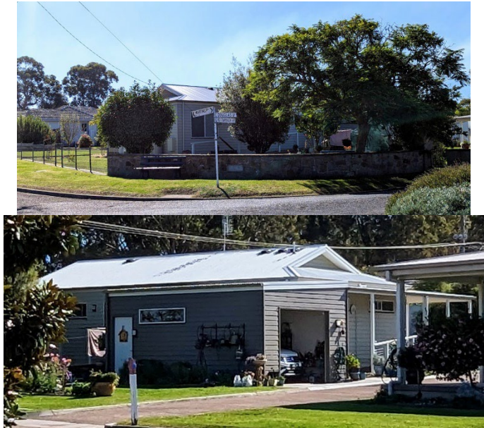
Some major works and more needed...
